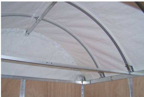
Interior, showing roof bow system. White color allows light penetration.
