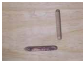
Close-up of pre-cut fastener slots
